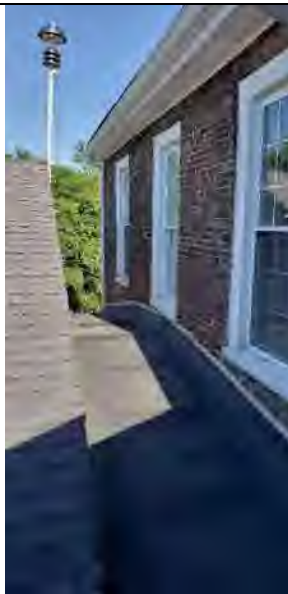
Photograph 3: North West Structure looking west.
