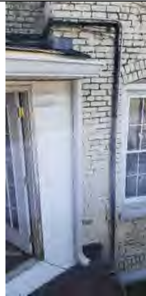
Photograph 8: North east structure looking east.
