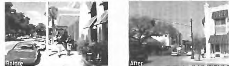
Park Avenue, Winter Park Florida. Travel lanes was narrowed, sidewalks widened, sewer lines replaced, and communication lines added. The redevelopment of the street was paid with by a combination City Funds and a Bond Fund.
