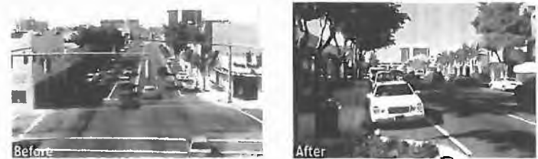
Sunset Drive, South Miami Florida. A travel lane was removed, sidewalks widened and drainage improved. The redevelopment of the street was paid for by the developer who was building new mixed use buildings on the street.
