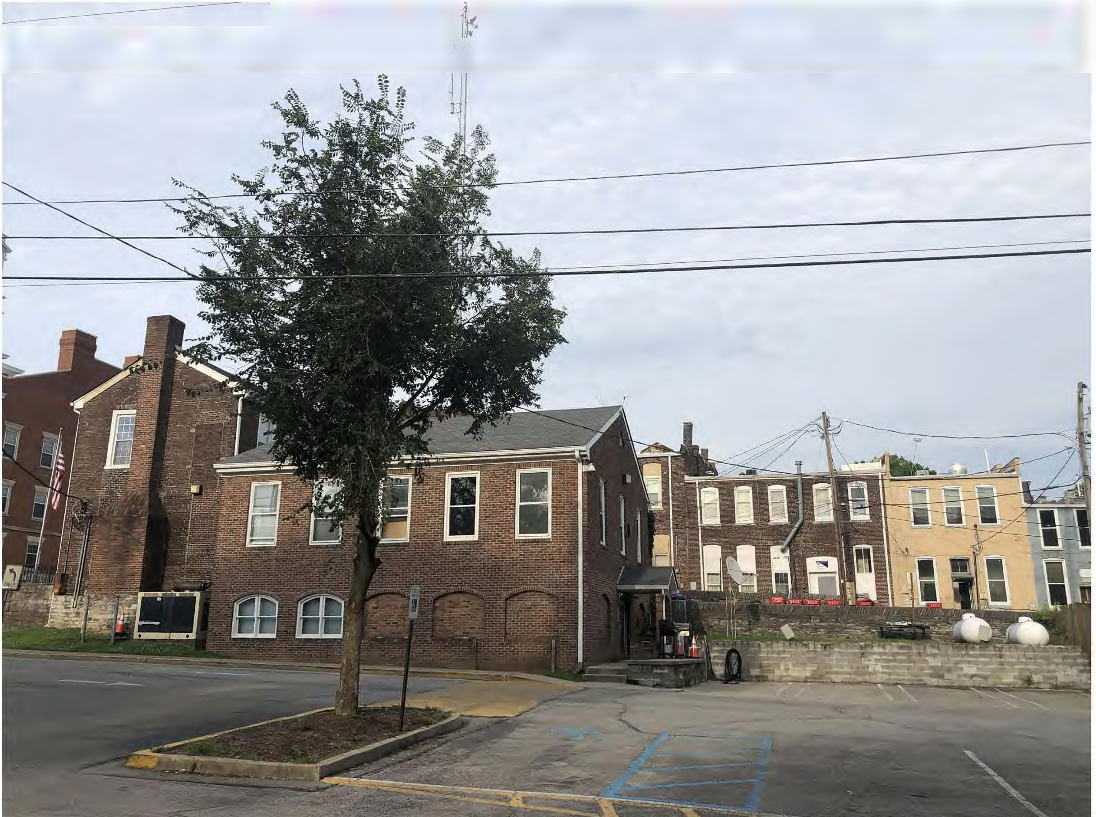
Existing Police Station - side elevation (facing park)
