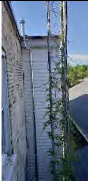
Photograph 1: South East Addition looking south.
