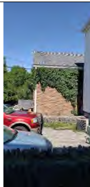
Photograph 24: South addition looking west.
