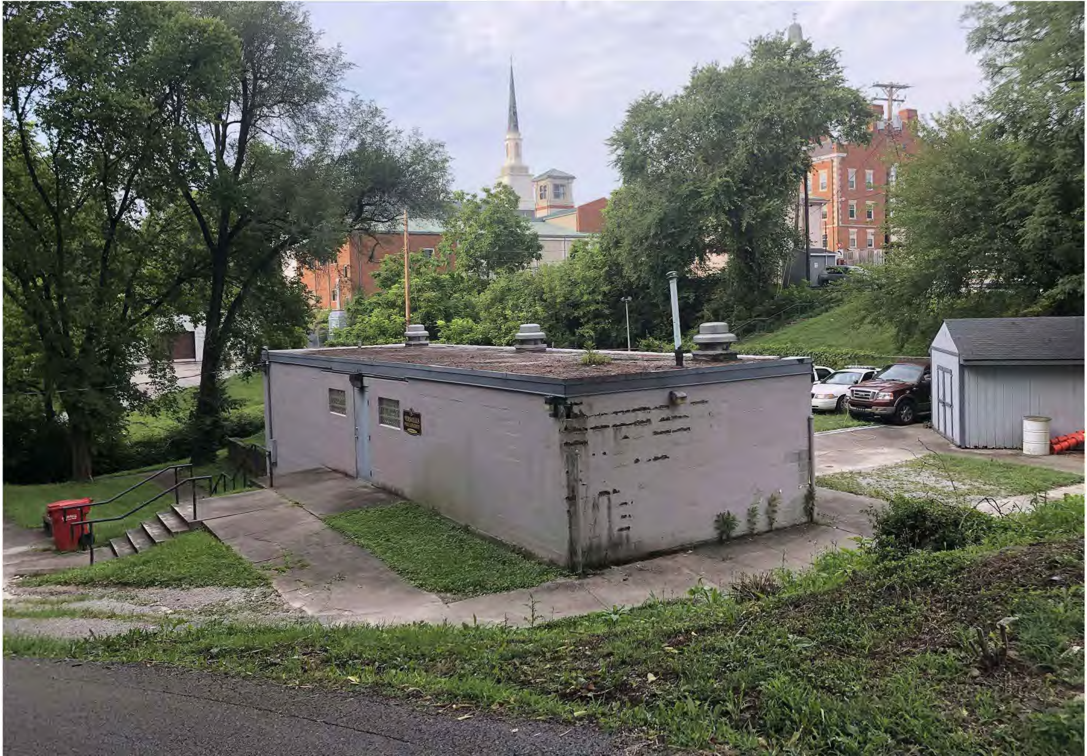
Existing Police Holding Station - rear elevation (at park)
