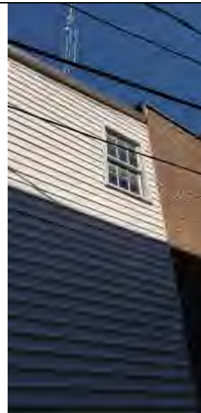
Photograph 12: South east structure looking west
