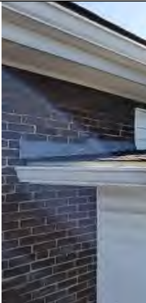
Photograph 7: North east structure looking east.
