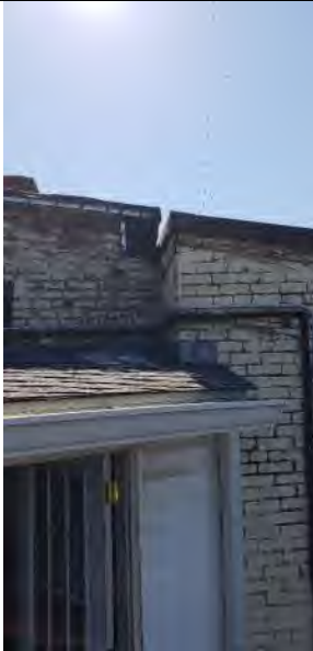
Photograph 5: North east structure looking east.
