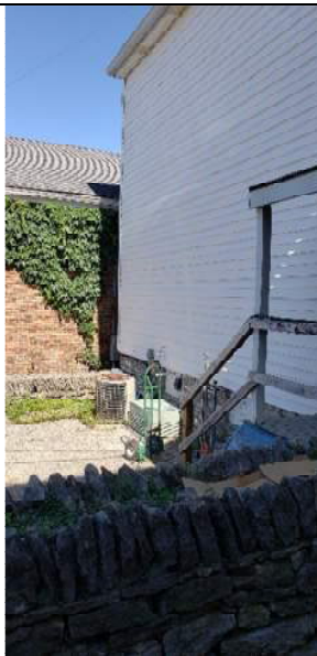
Photograph 11: South east structure looking west
