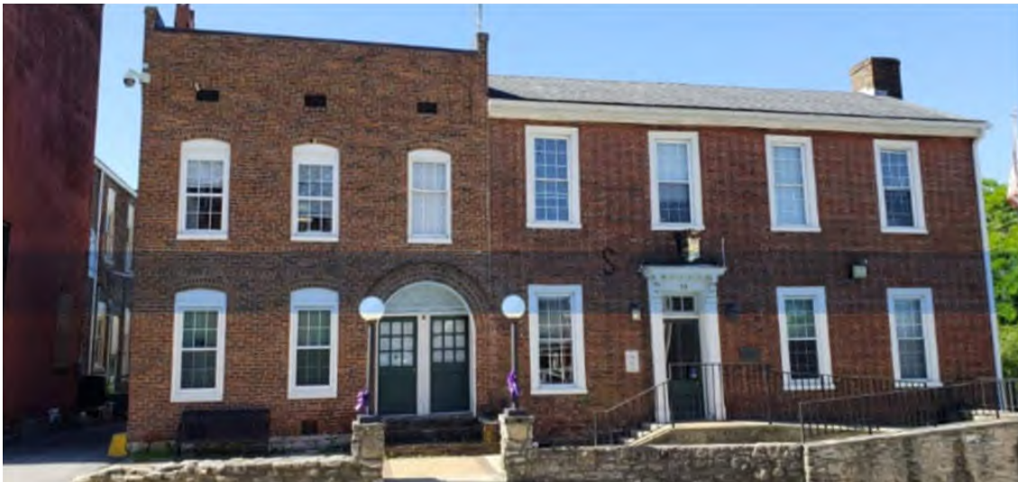
FORMER POLICE BUILDING
