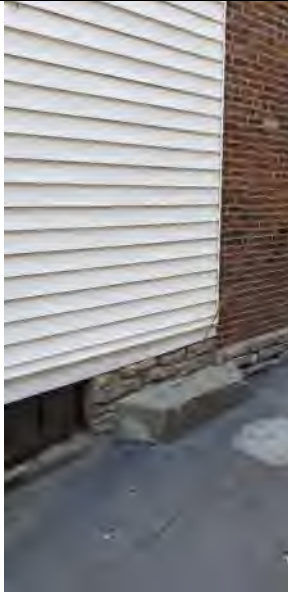
Photograph 13: South east structure looking west
