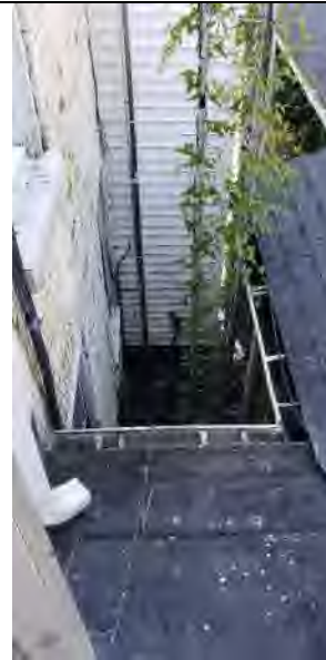
Photograph 2: South East Addition looking south.
