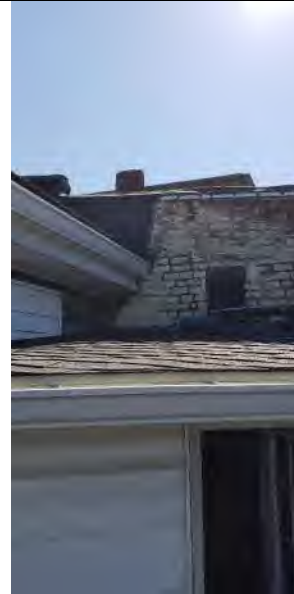
Photograph 6: North east structure looking east.
