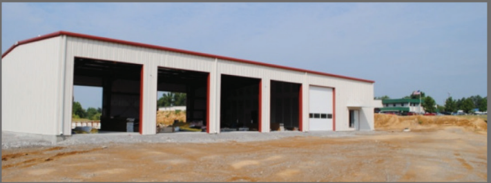
CRITTENDEN COUNTY FIRE STATION
