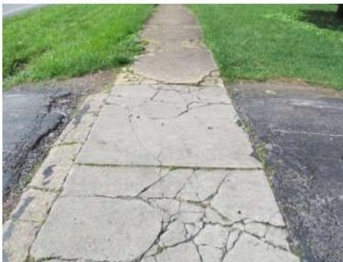
**Figure 3** - Broken walk to be replace on S. Columbia Ave.
